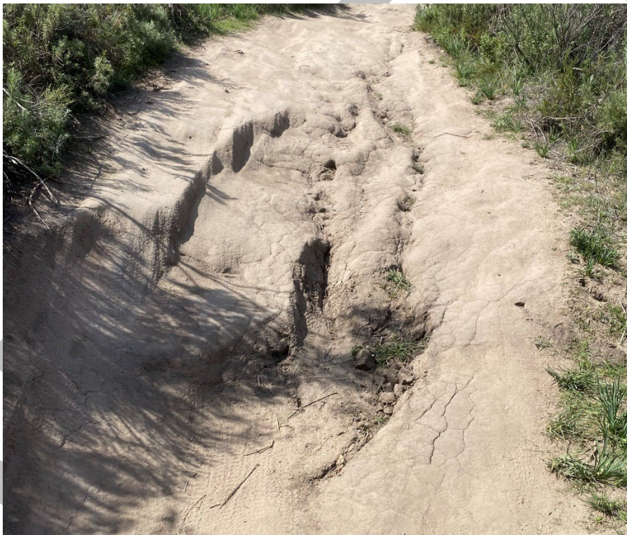
Figure 3: Trail widening. This trail was originally approximately 3 feet wide. As incision developed, trail users began avoiding the eroded tread, trampling adjacent vegetation and progressively widening the disturbed corridor.
