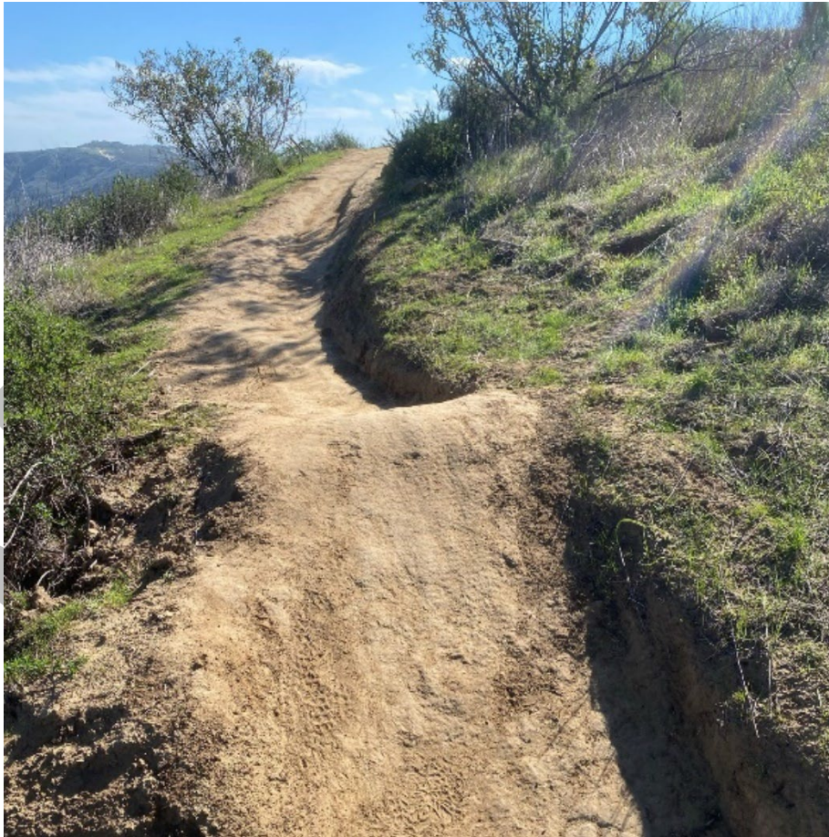
Figure 9: Constructed features, such as the jump shown here, often indicate that the trail is a purpose-built trail.
