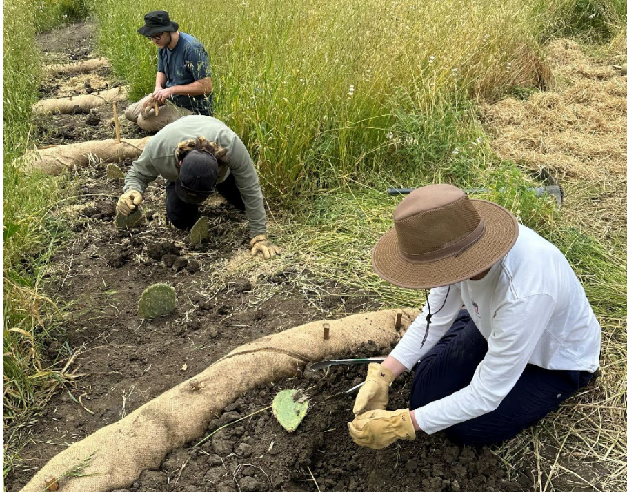
Figure 22: Tasks such as installing straw wattles and planting cactus are well suited for volunteer work.
