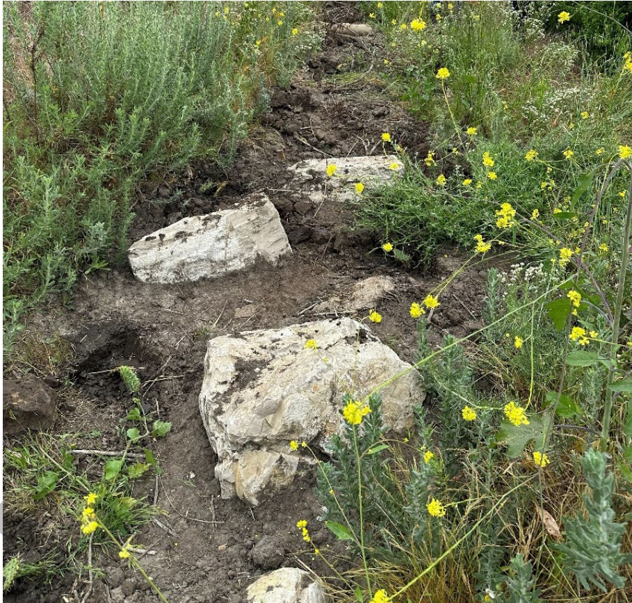
Figure 14: Rock “gargoyles” should be spaced closely enough to prevent easy weaving by bicycle and embedded deeply enough to make removal difficult.
