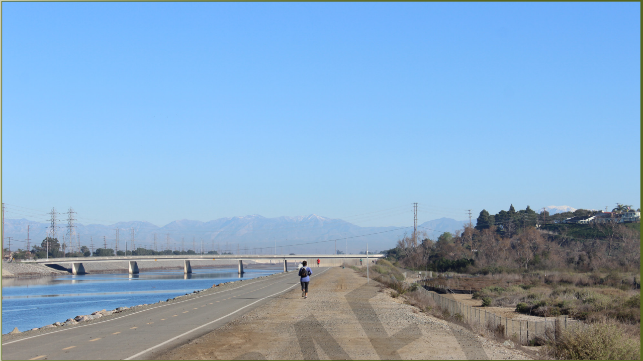
View of the Banning Channel Bikeway adjacent to TARE, and the Santa Ana River Footbridge, which provides an important connection to greater Orange County via the Santa Ana River Parkway.
