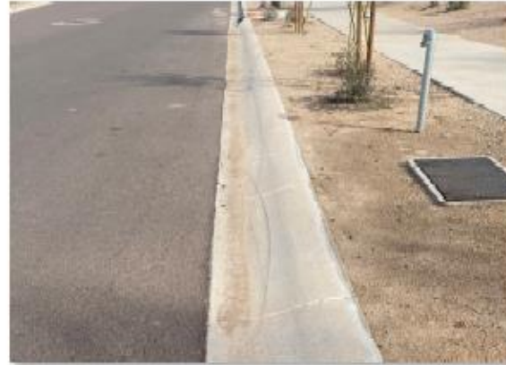
Concrete Rolled Curbs
