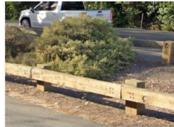
Rustic Wood Railings
