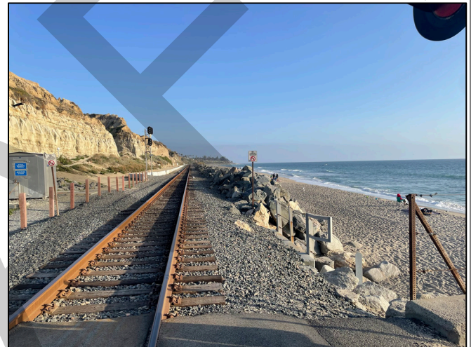
LOSSAN Railroad with riprap (Anchor QEA, March 6, 2023)
