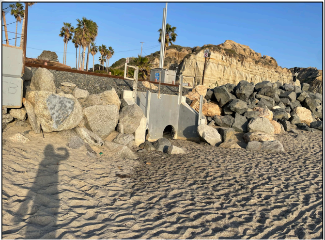
Stormwater infrastructure at Califa Beach Park (Anchor QEA, March 10, 2022)
