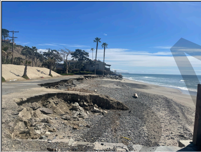
Capistrano Beach Park adjacent to Capistrano Bay District (Anchor QEA, March 6, 2023)
