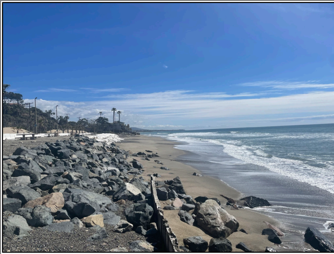
Capistrano Beach Park riprap and sandbags (Anchor QEA, March 6, 2023)
