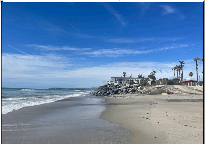
Capistrano Shores from North Beach (Anchor QEA, March 6, 2023)
