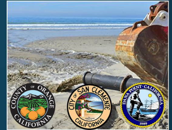
Regional Beach Sand Project III
