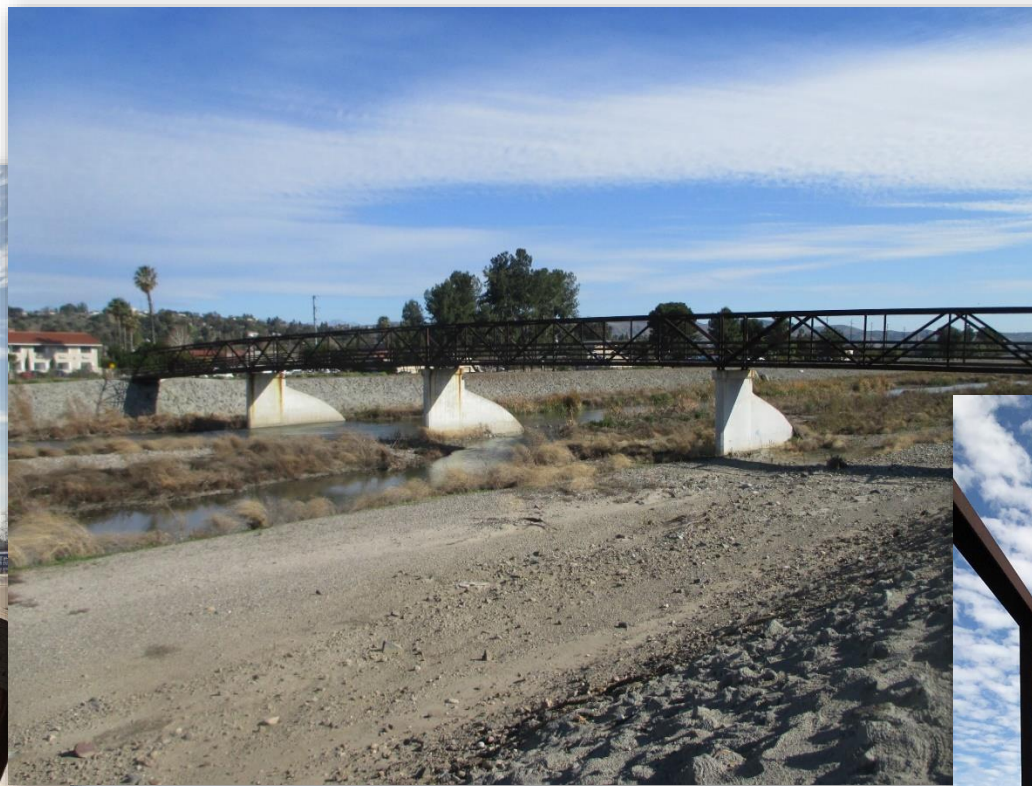
Bridge #2 – Santa Ana
