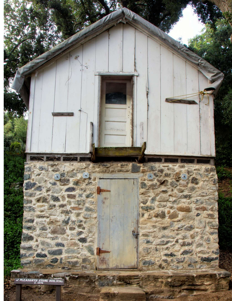
After first floor restoration
