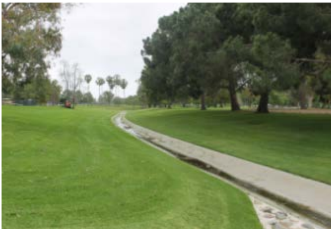
Mile Square Regional Park- Drainage Channel, 2019
