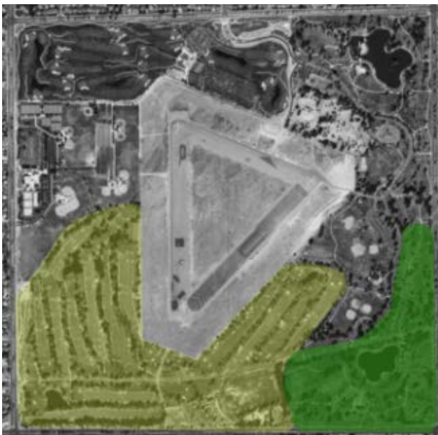
1970 - Mile Square Regional Park Phase I construction complete
