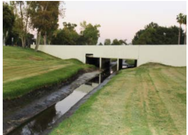
Existing Drainage Channel and Circulation Bridge
