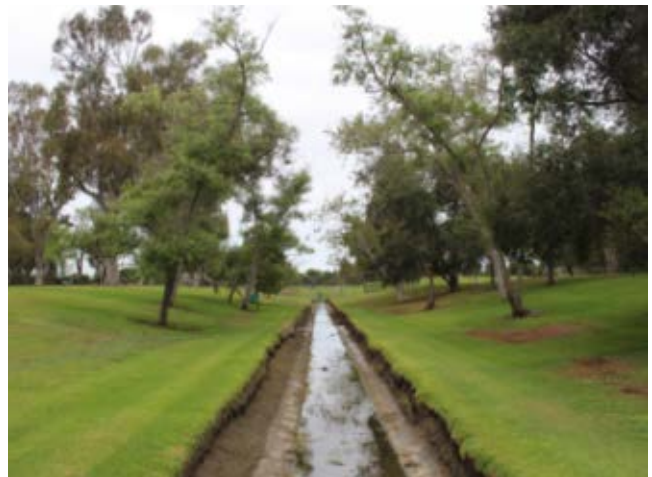
Mile Square Regional Park - South Storm Drain, 2019
