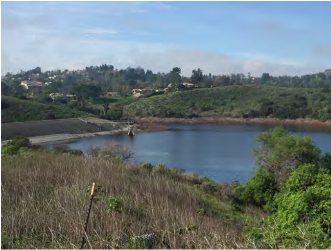
Existing Peters Canyon Dam Outlet Tower
