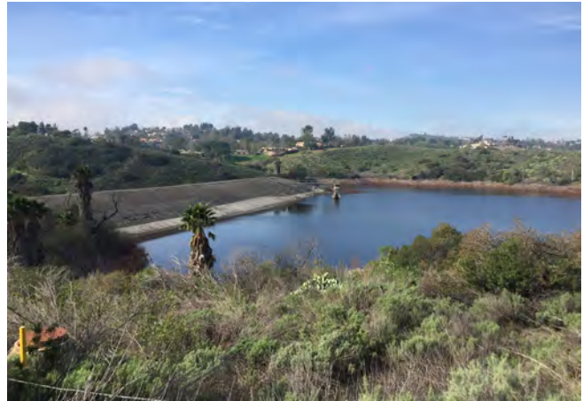
Peters Canyon Dam – 2017
