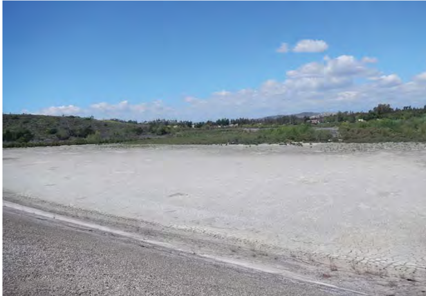
Photo 5: Looking northwest from the UPCR dam into the reservoir (currently dry)
